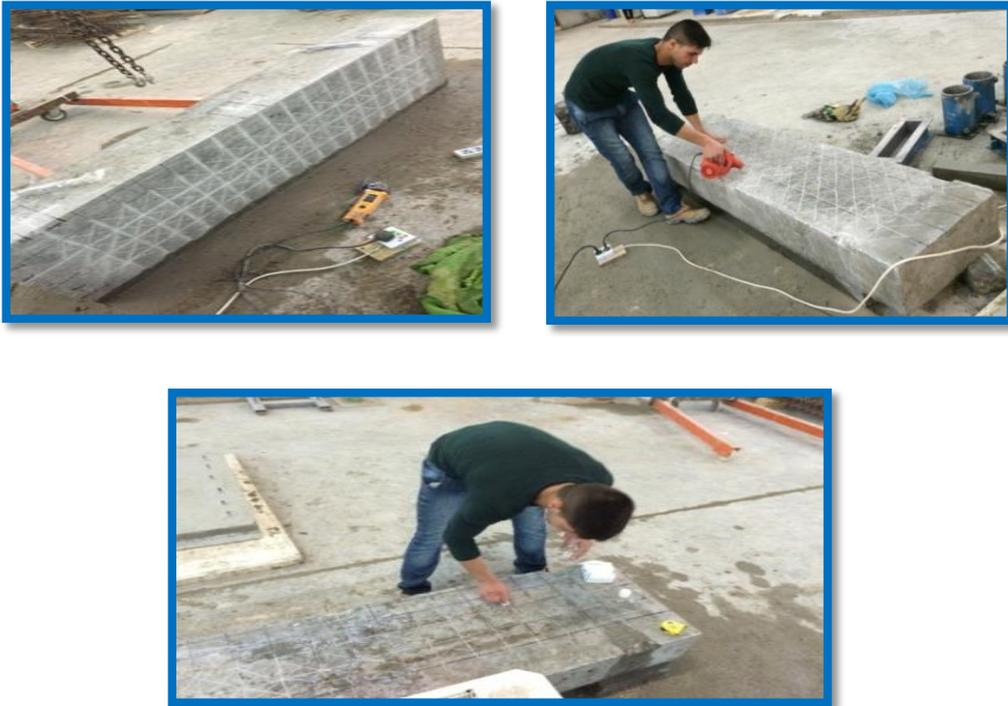
Fig. (4): Concrete surface preparation
