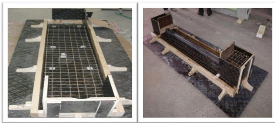
Figure (2): Reinforcement of composite steel tube concrete beam specimen.
