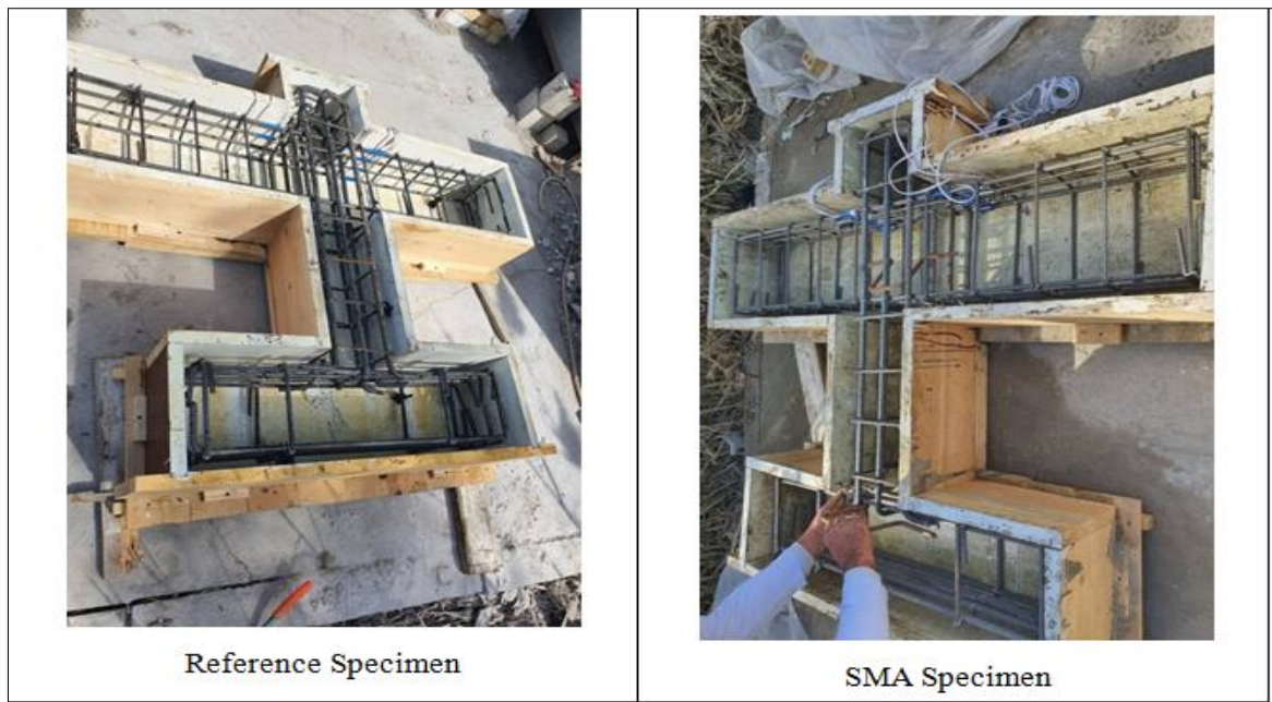
Figure 6. Steel reinforcement of testing specimens
